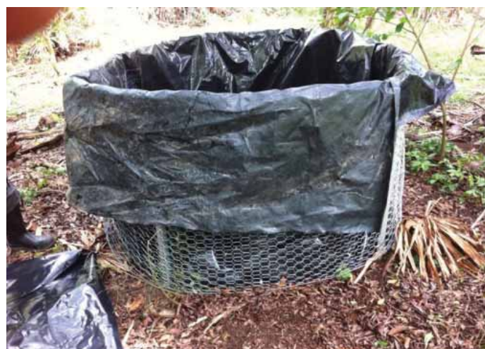
Figure 3: Interior lining of black plastic extending over the top of the structure.
