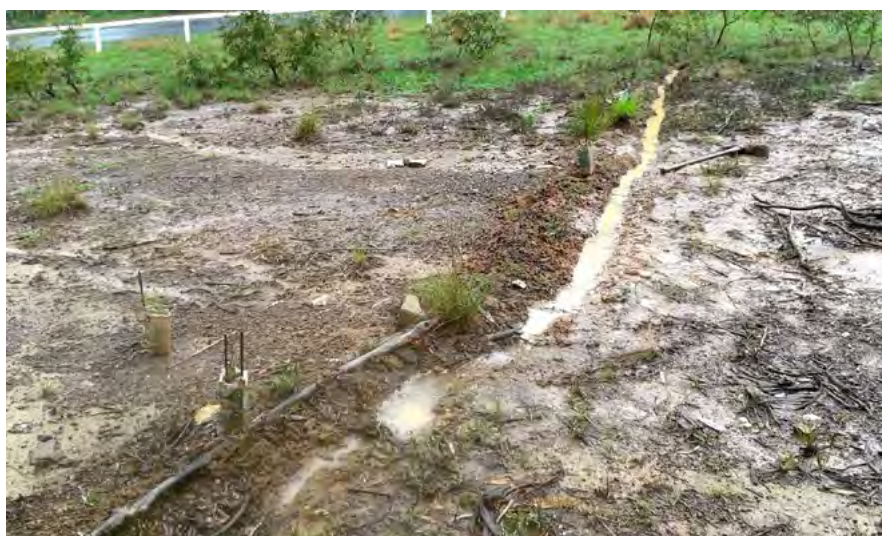
Left: Diverting water off route up Mt Mutton, Uralla NSW.
