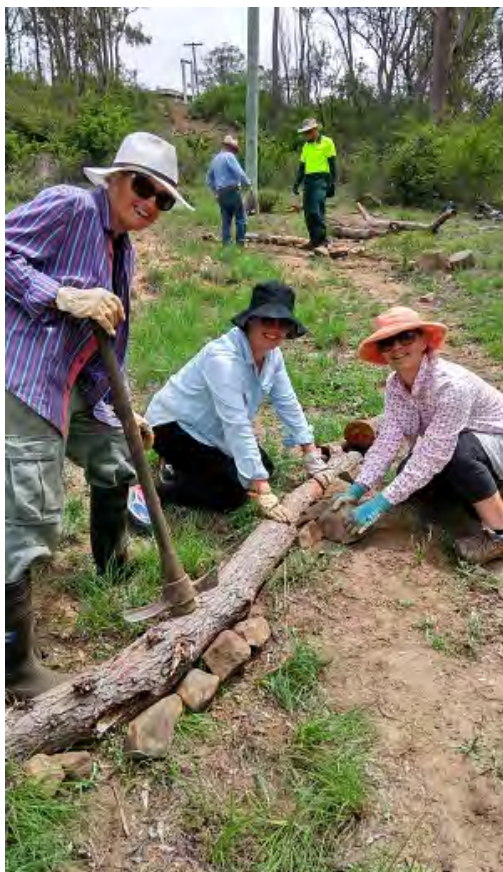
Left: Diverting water off route up Mt Mutton, Uralla NSW.
