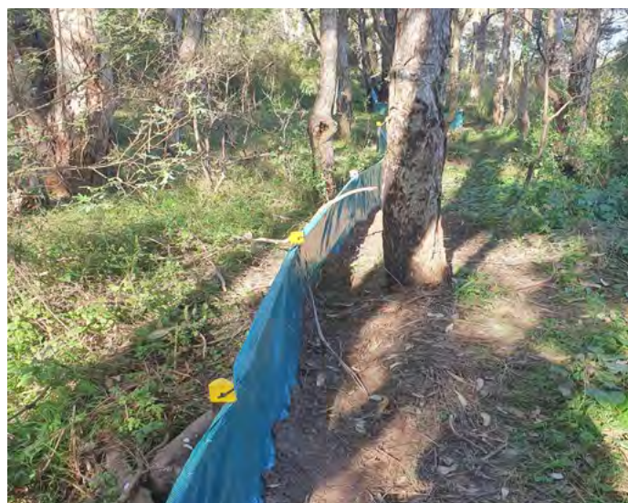
The sediment fence to minimise weed dispersal Photo Sue Pritchard
